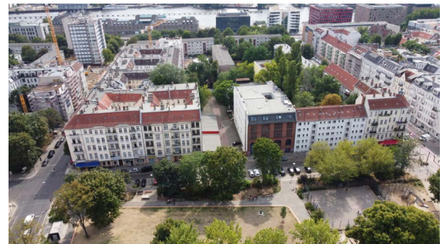
Aerial view of Rudolfplatz substation ©Linus Krueger
